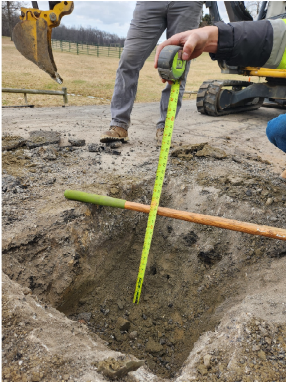
Figure A-3: Excavation in Dinninger Road
